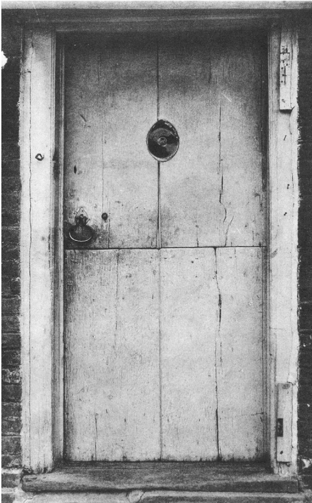
Figure 4.2: Exterior side of the sash batten Dutch door on the Hendrick Kip House in Dutchess County (adapted from Reynolds 1931: Plate 1 on an unnumbered page). The glass peep hole is called a “bull’s eye” in Reynolds’s book. The two leaves of the door have two vertical boards on the exterior.
