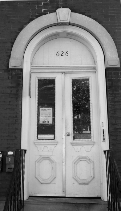
Figure 4.18: Front door from the first phase on a row house.
