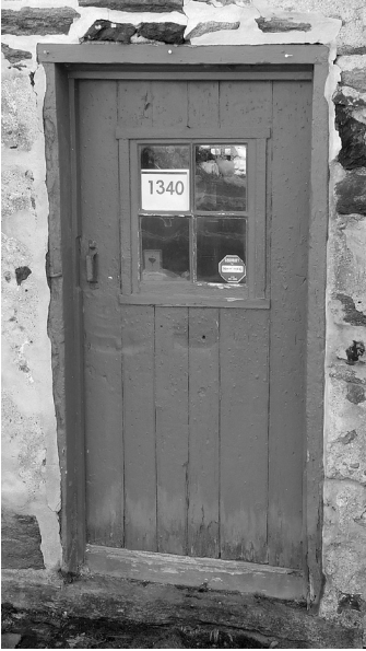
Figure 4.4: Sash batten door on the blacksmith shop in Marshallton, Pennsylvania.
