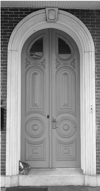
Figure 4.16: Very stylish Front door on a Second Empire style house in Pottstown, Pennsylvania with its original casing and keystone. This door features tear shaped lights at the top, decorative panels accompanied by pressed wood motifs, and concentric circle motifs.
