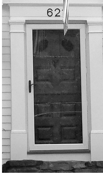
Figure 4.7: Primary entrance of a Federal style house near Somerville, New Jersey. The oval lights in the frieze panels are installed diagonally.
